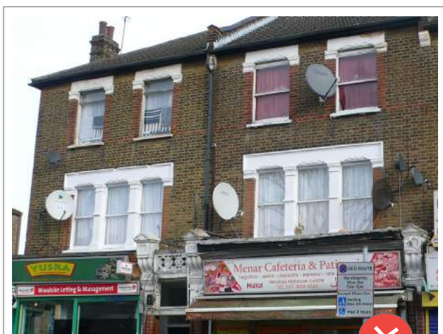
Satellite dishes shouldn't usually be mounted on the front of buildings
