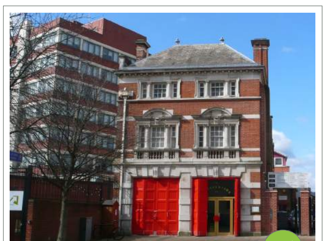
Change of use can result in the long term preservation of a listed building as in this example in the Tottenham Green Coconservation Area
